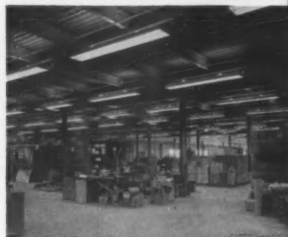
"BI-FLO UPLIFTER" 72% downlight — 28% uplight, provides greater seeing comfort for industrial areas such as Assembly Lines.
